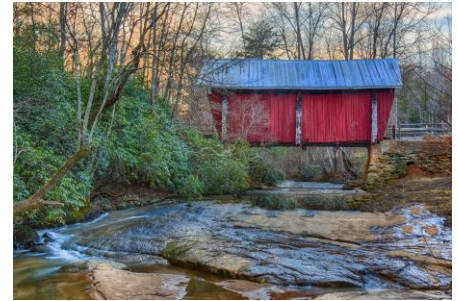
Campobello's covered bridge along the South Pacolet River, the last one in SC
